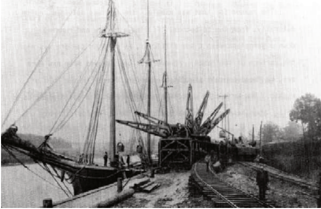
Early machinery for loading and unloading ore — 1880. The unloading devices are “Whirleys” which replaced the Irish man with a wheelbarrow.
