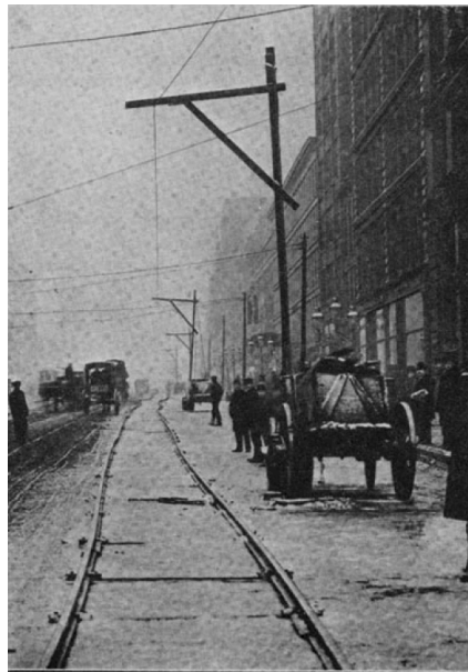
“The night of December 26, 1906, the Forest City Company attempted to lay temporary tracks on top of the pavement on Superior St., N.W.”
