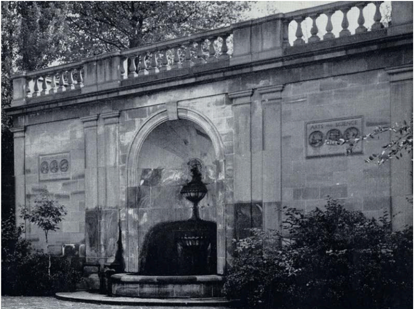
Lower Terrace Wall of the Italian Cultural Garden
